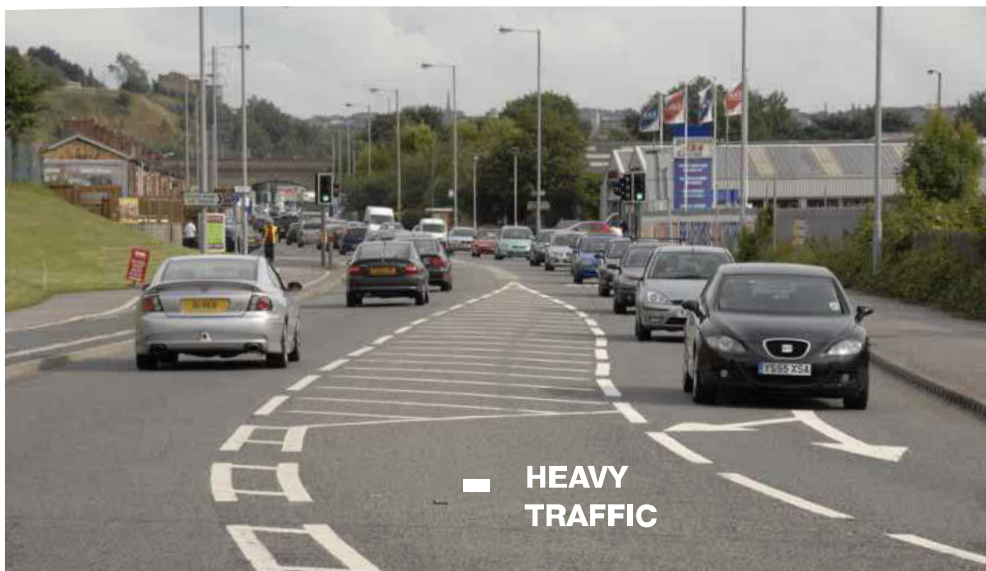
View down Canal Road
