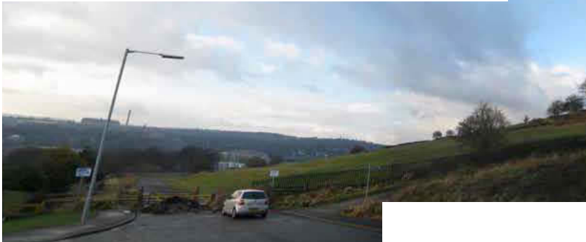
View down Poplars Park Road
